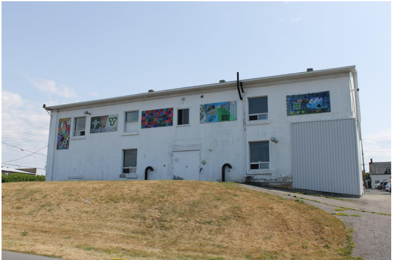
Picture of Alexandria Water Treatment Plant prior to renovations
