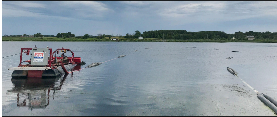
Figure 4. Dredge in a lagoon cell.
