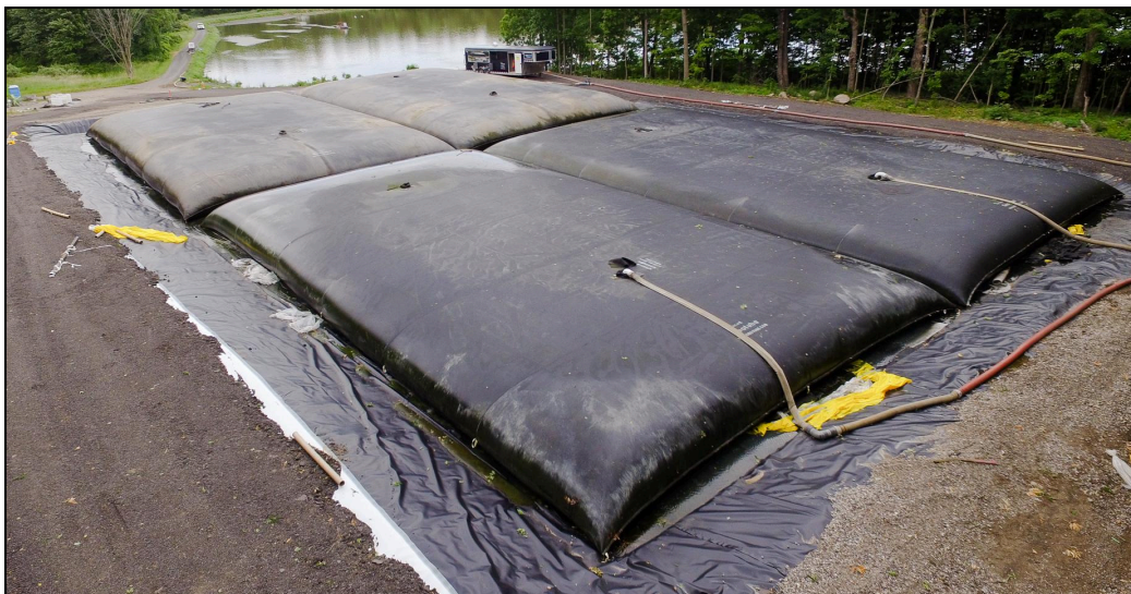
Figure 3. Geotube® dewatering cell constructed using impermeable liner, non-woven geotextile and GFF (GFF is under Geotube units, not visible).
