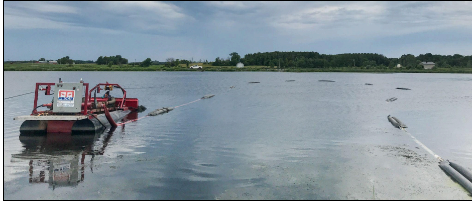
Figure 4. Dredge in a lagoon cell.
