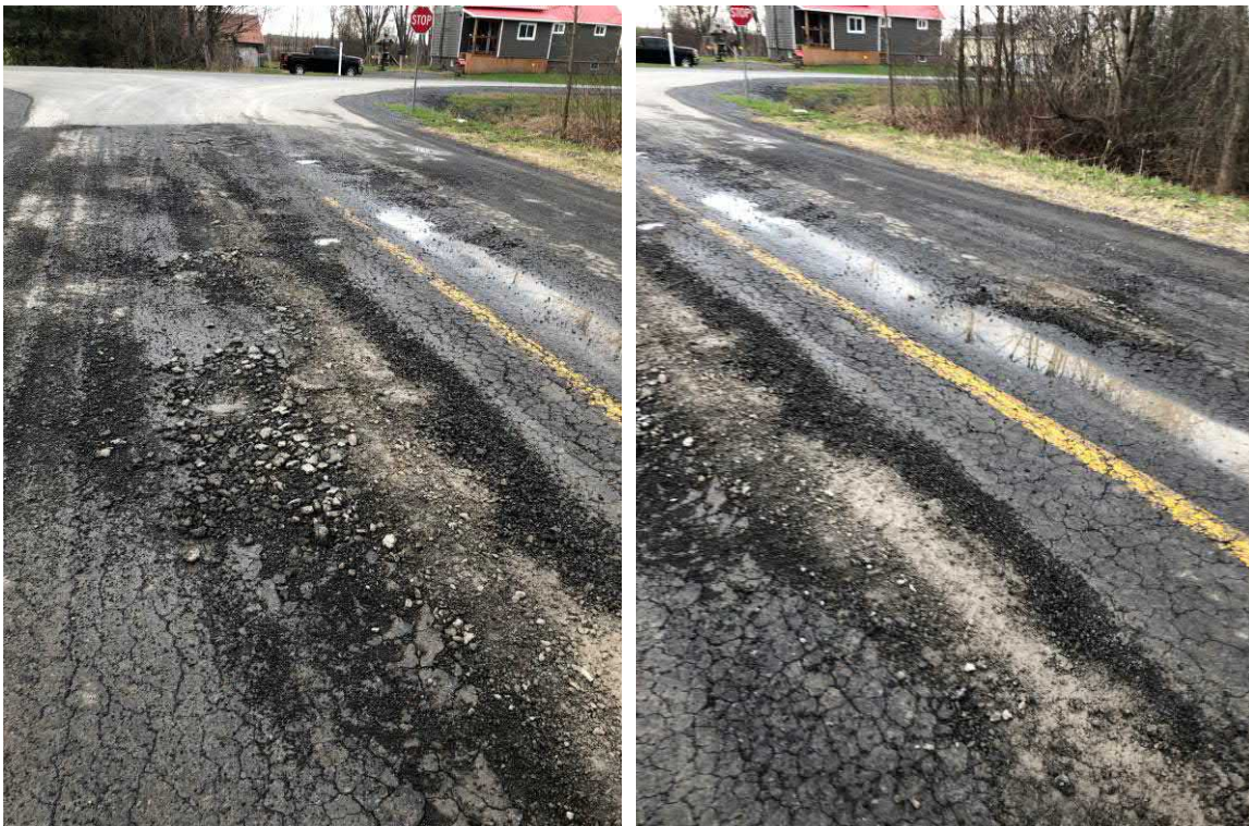
Figure 4.10.1: Location J, Severe Frost Heave
