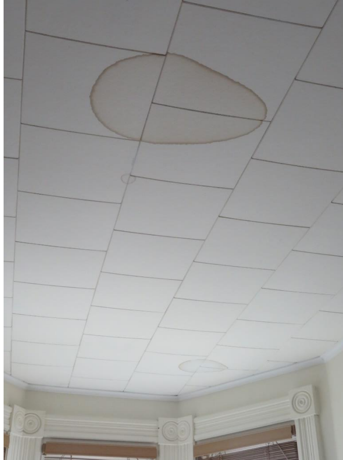
Ceiling of Front Bedroom – Water Damage
