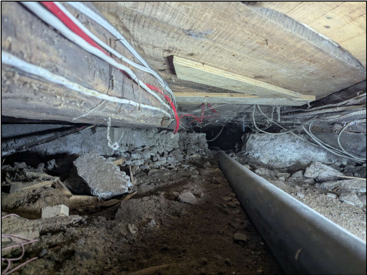
PHOTO - EXISTING CRAWL SPACE CONDITIONS
