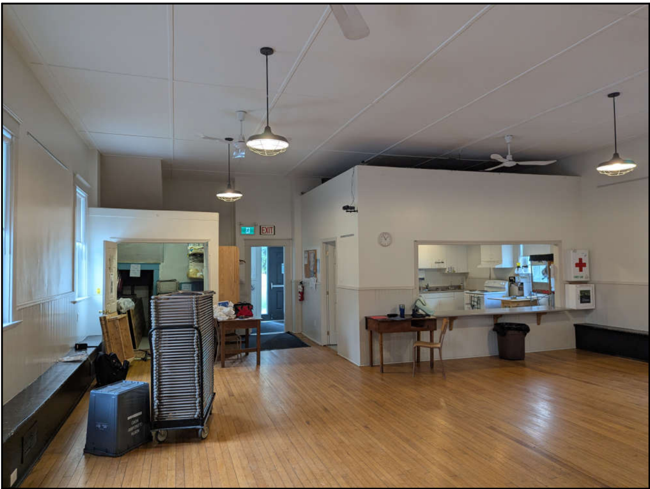
PHOTO - EXISTING INTERIOR PARTITIONS
