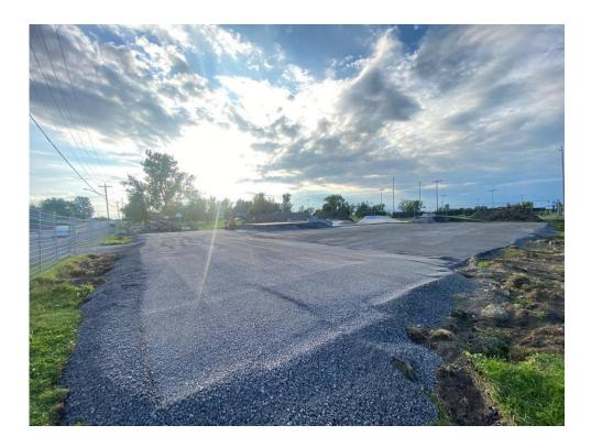
On September 19, 2023, the workers from Papillon Skateparks started the first phase which involved the setting of grade stakes with levels and strings to create proper drainage and prevent standing water on the slab. The second phase involved the laying of the forms for the flat ramps, quarter-pipes, A-Frame, handrails, boxes, ramps, stair sets, banked ramps and flat launch/rest areas.
