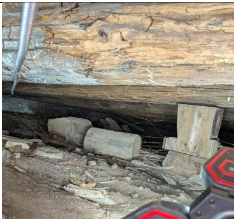
FIGURE 11: Makeshift Timber Post
