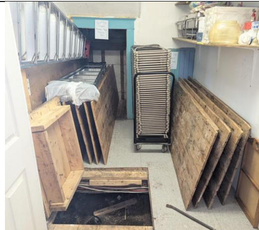
FIGURE 4: Storage Room and Floor Hatch
