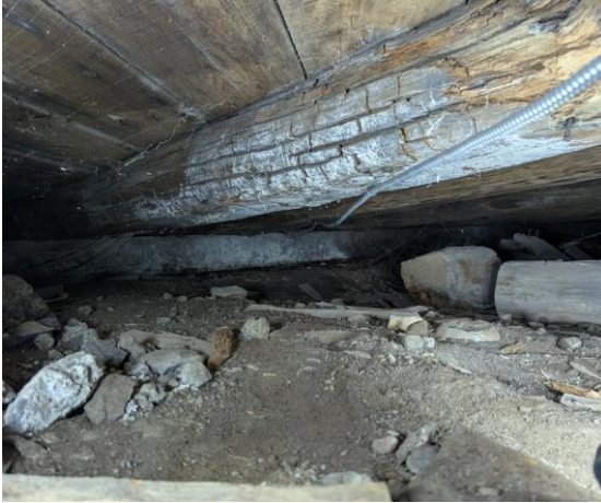
FIGURE 9: Timber Beam Rot
