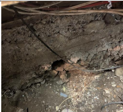
FIGURE 5: Honeycombing
